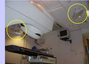
Figure 1. AlignRT cameras mounted to the ceiling in a linac room.
